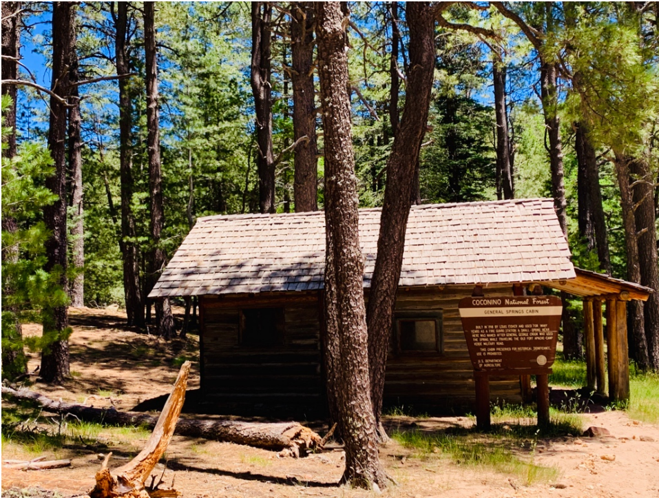
General Springs Cabin as you complete the Fred Haught Trail and head up the dirt road to the Rim Road
